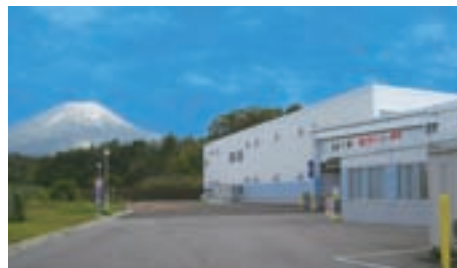
▲ The expanded warehouse adjacent to the Daisen Production Plant
